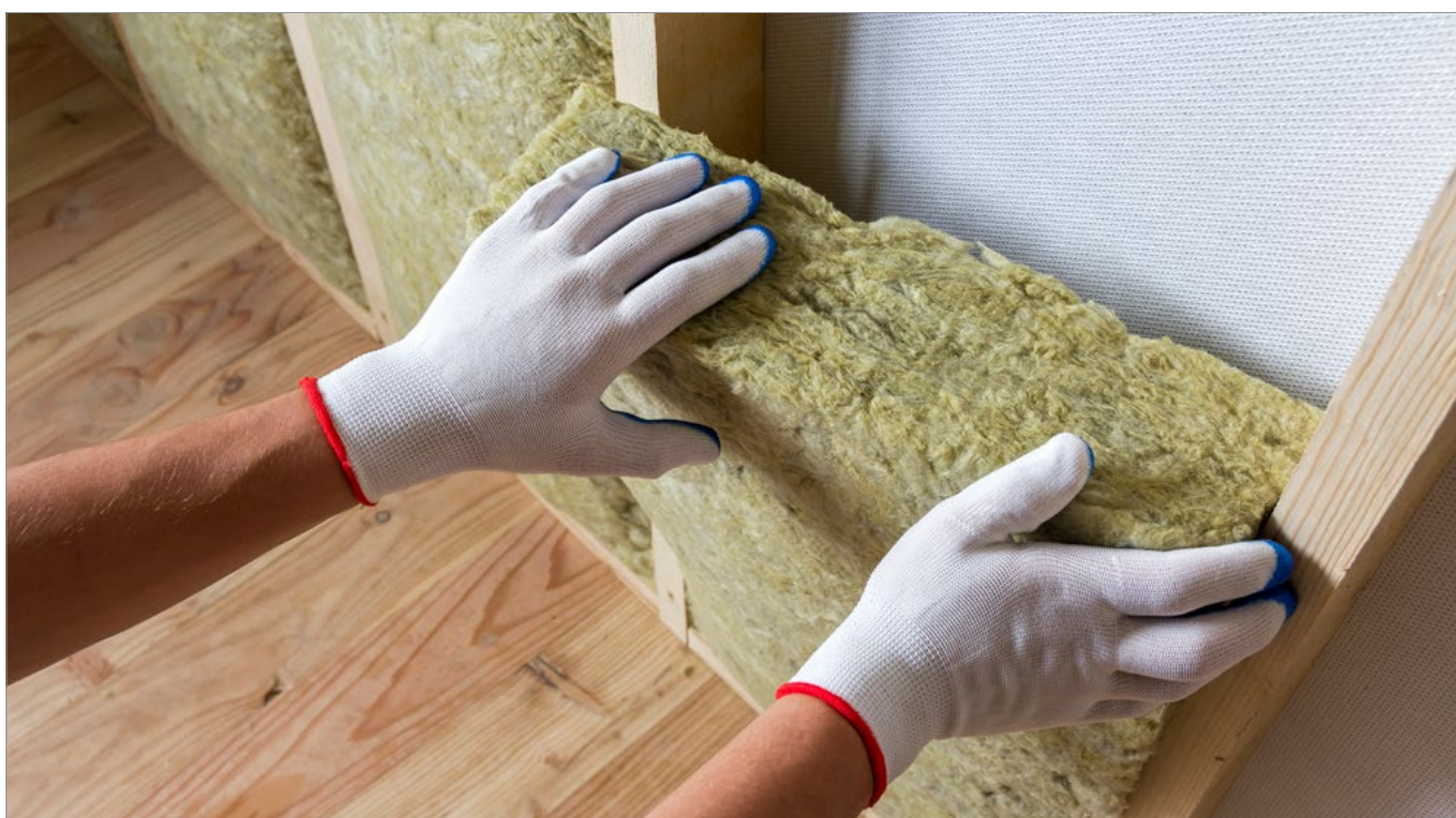
Insulation must be installed with no gaps, folds or compression.
